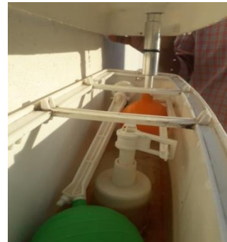
Mechanical Cylinder and Piston based Toilet Liquid Sanitizer Dispenser (February 2021)
